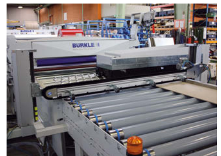
Heizzone zur Plattenvorwärmung Heating zone to pre-heat the boards
